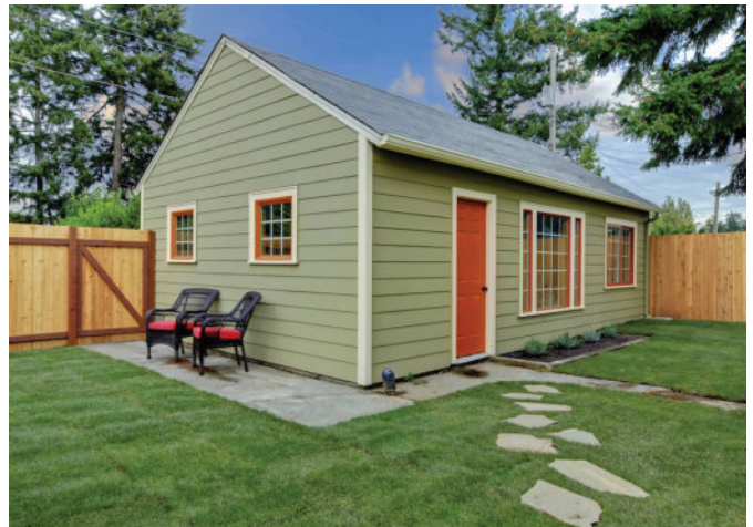
Garage to ADU: A detached garage was converted into a living space for the owner's parents.
